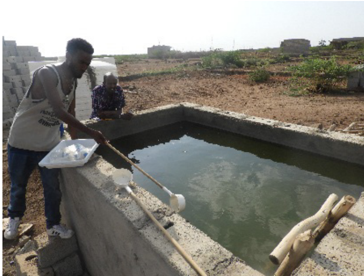
Figure 2b. Concrete cistern in Ethiopia
