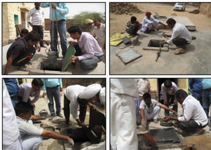
Figure 6a. Community training/demonstration of mosquito proof lid replacement on underground water tanks “tankas” in India”
