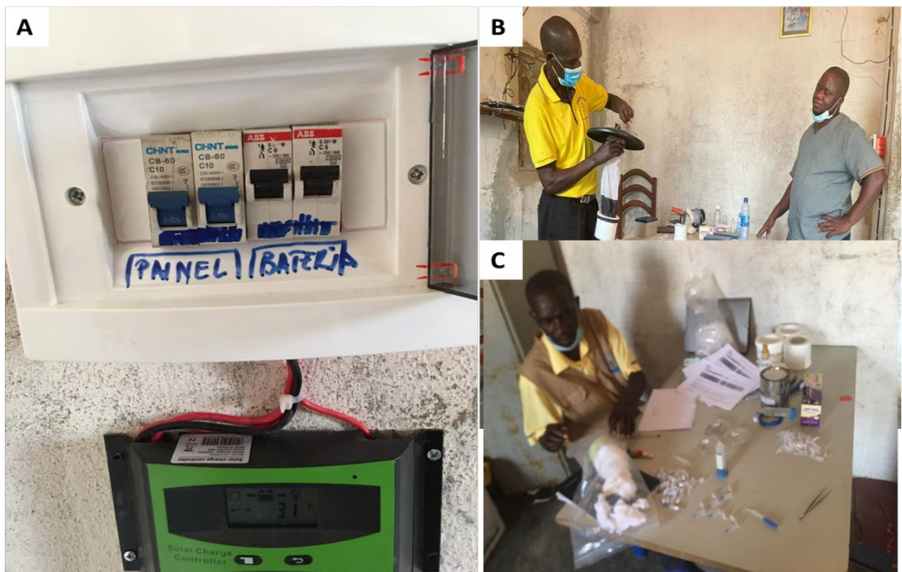
Figure 2: Photograph of the Solar Panel Charging System for CDC LTs in Mulundu Village, Huambo Province (A), Community Collector Demonstrating Retrieval of Mosquitoes from a CDC LT as VectorLink Technician looks on (B), Anopheles Mosquitoes from CDC LT Stored Individually for Molecular Analysis (C)
