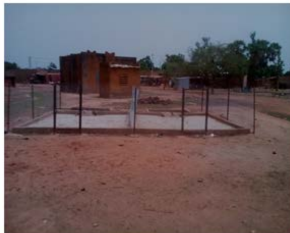
Figure 8: Standard IRS Site with Washing Slab, Soak Pit, and Water Reservoir
